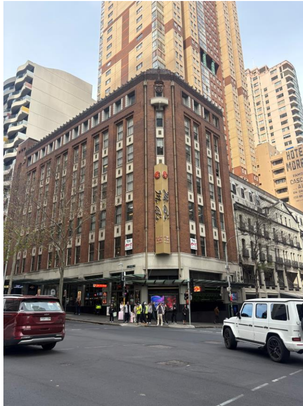
Figure 1: 390-396 Pitt Street, Haymarket, viewed from the north-west
