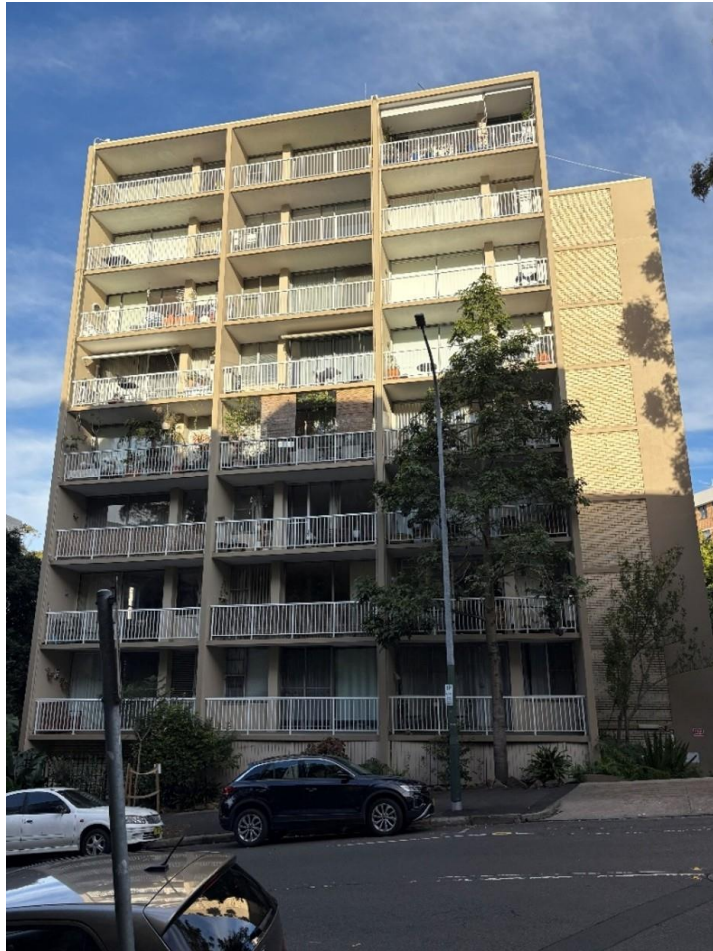
Figure 1: 74-76 Roslyn Gardens, Rushcutters Bay viewed from the south
